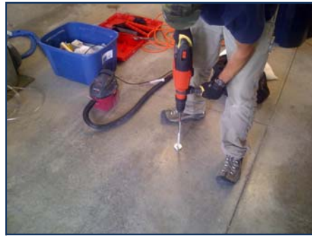
Installation of a soil vapor sample point.
